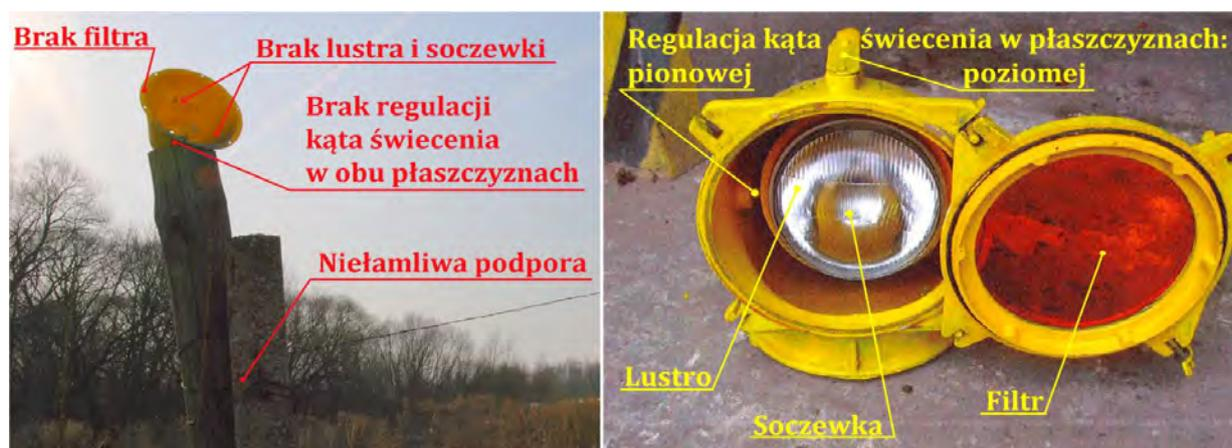
Photo 23. Comparison of lamps of the lighting system
